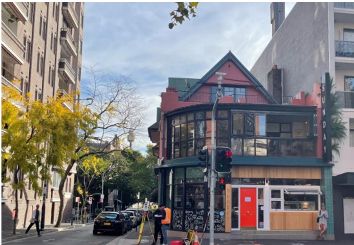
Figure 2: Front of site (eastern elevation) viewed from Macleay Street
