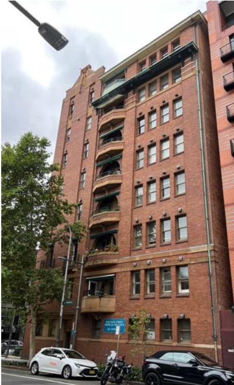
Figure 6: View facing north-east, locally listed heritage building at 1 Greenknowe Avenue known as Kingsclere (1585), located south-east of the subject site
